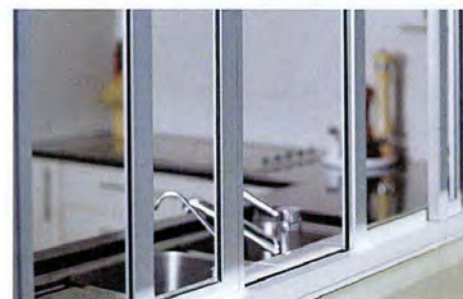
6. WINDOW / DOOR FRAMES (GF) - Clear anodised aluminium
