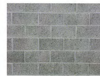
10. HALF HEIGHT BLOCKWORK (BLK)
