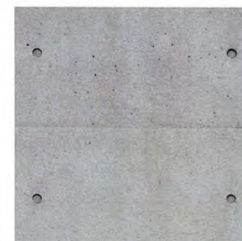
4. CONCRETE COLUMN / SOFFIT - Off Form Concrete finish
